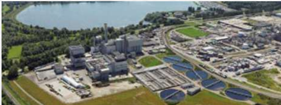
Dordrecht: wwtp & sludge incinerator
